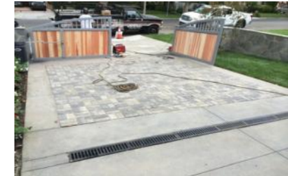
Permeable Paving (w/ 1' – 2' sub base)
