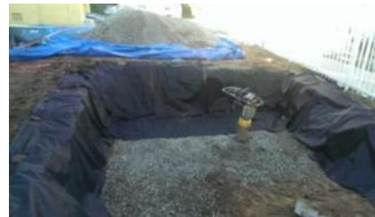
Permeable Paving (w/ 1' – 2' sub base)
